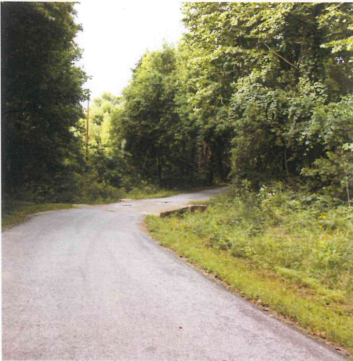
VIEW OF BRIDGE FROM OLD WIRE CONSERVATION PARKING LOT
