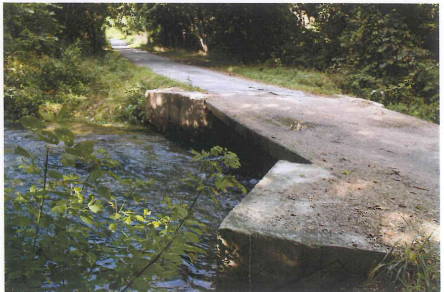
VIEW OF NORTHEAST SIDE OF BRIDGE
